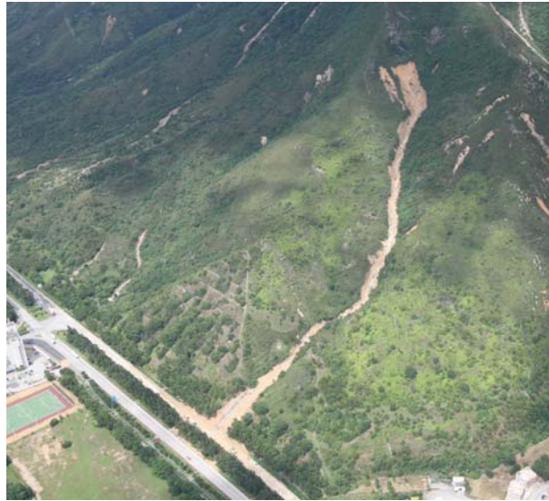
Figure 12: Debris flow affecting a road with low traffic density
